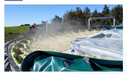
After years of operation sulphur nets can become laden with sulphur which reduces the effectiveness of the net to capture sulphur and could lead to net and internal tank damage. Marches Biogas can offer the safe and effective cleaning of a sulphur net, together with any necessary repairs. During the clean our engineers also inspect the internal top section of the tank including centre column and biogas pipework, clean any viewing windows and service the pressure relief valves.
